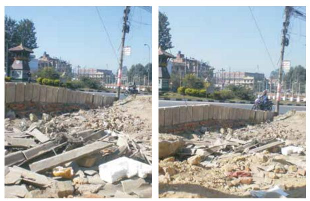
Figure 19.Asbestos Waste dumped at Maitighar Mandala, water recharging zone, the only underground reliable source of drinking water for capital people of Kathmandu (November 2013)
