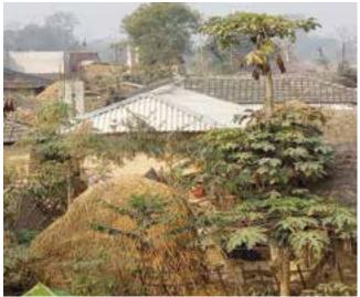
Figure 2 A typical residential house in Terai with traditional Clay soil tile, Asbestos sheets and concrete roofing together
