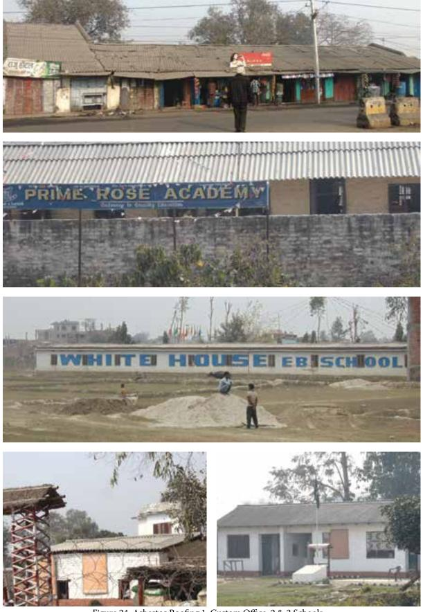
Figure 24. Asbestos Roofing 1. Custom Office, 2 & 3 Schools , 4. Custom Security Office, 5. Security Guard Quarters
